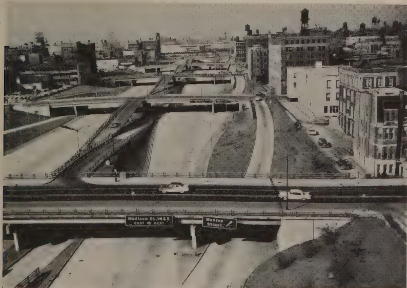
239 Chicago. A depressed freeway skirting the downtown area. Note the great scale of the construction, how the local roads flow over the freeway, and the frequency of the access ramps which are about as close as could reasonably be contrived. The down-grade of the 'on' ramp assists acceleration, and the up-grade of the 'off' ramp helps deceleration.
